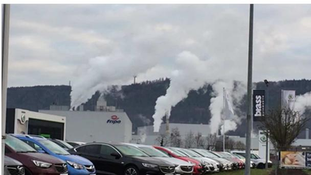
**Figure 2.** Wet steam emissions from a paper and cardboard factory. 1 m<sup>3</sup> of steam per second contains a thermal energy of 1.56 MW (Image: G. Muller).
